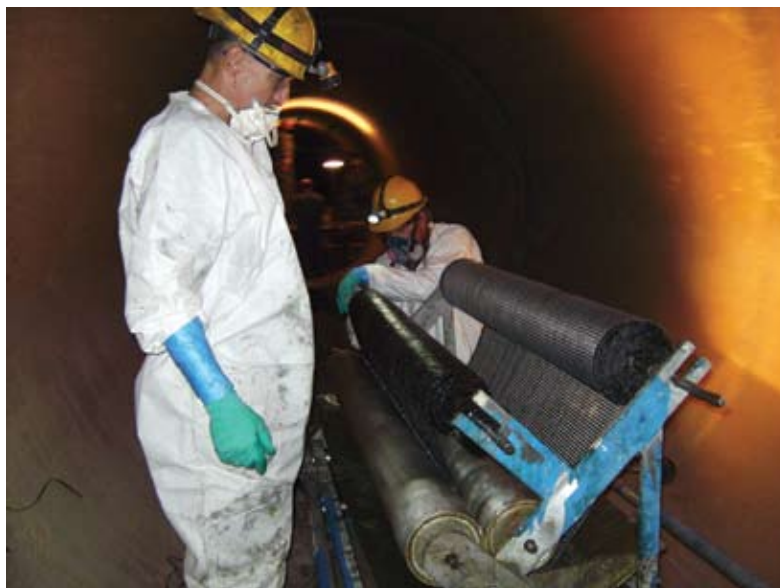
Saturating machine reassembled inside the pipe
