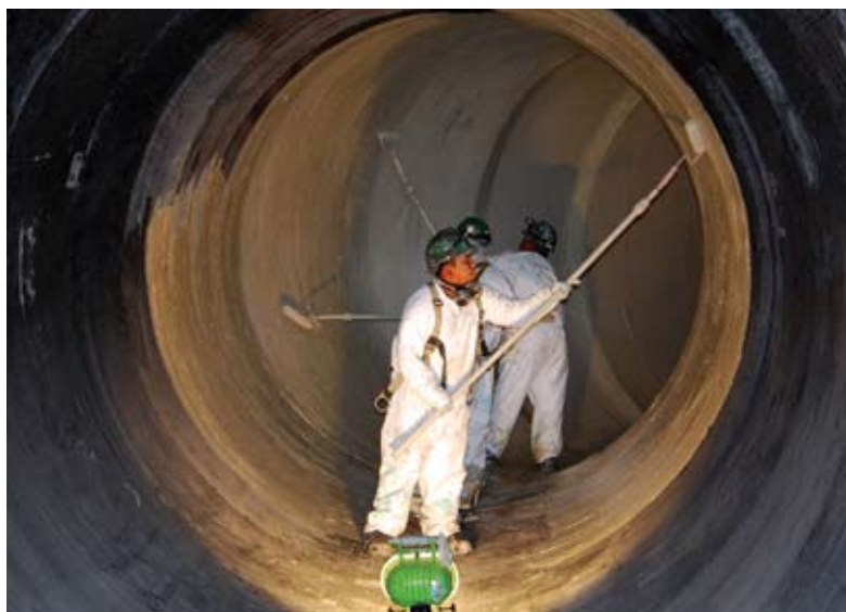
Application of final finish coating over installed FRP
