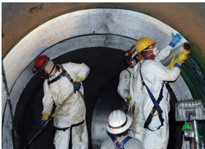
Installation of glass fabric on pipe
