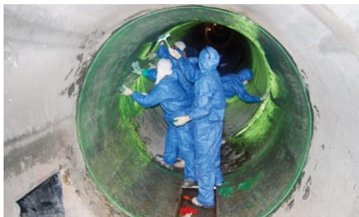
Fig. 6: Installation of FRP sheets on the interior surface of the pipeline
