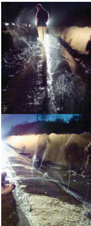
Fig. 2: Leaking after conventional crack sealing
