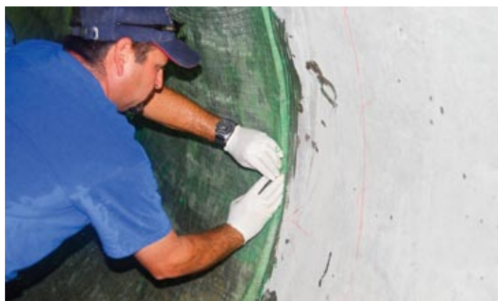
Fig. 7: Construction joint of FRP lining
