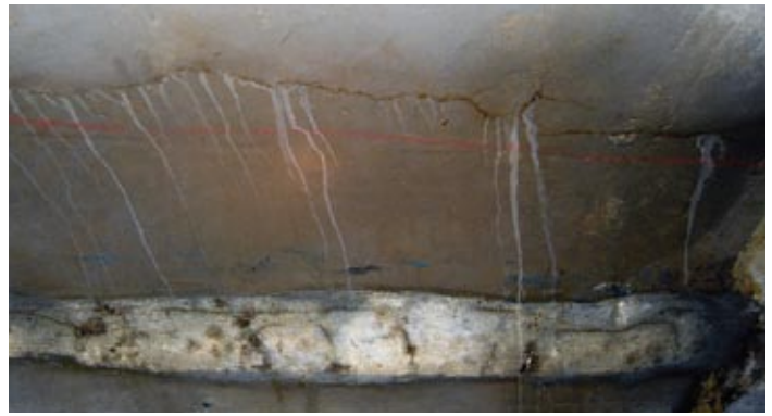
Fig. 3: Water seeping into pipeline
