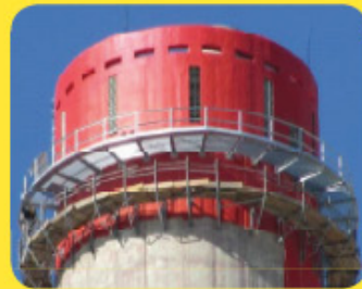
Restored chimney after repairs and painting
