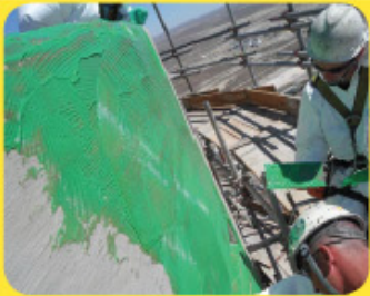
Application of tack coat
