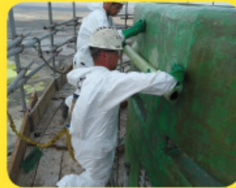
Installation of fabric
