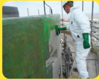
Application of tack coat
