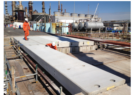
1 - Caltex Refinery Bridges
